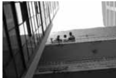
fig 10 Aiton Court courtyard, 2005
